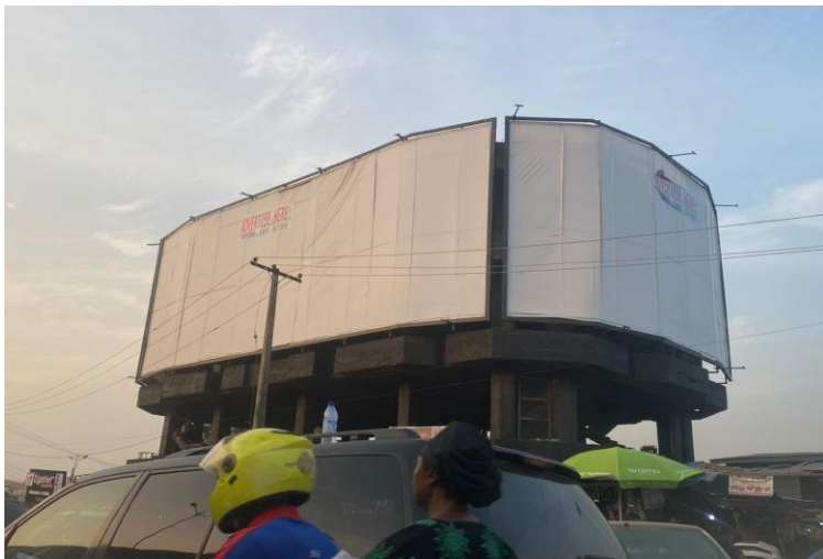
Plate 3: Abandoned Complex Building at Ita-Eko in Abeokuta. Source: Authors' Field Survey, 2024
