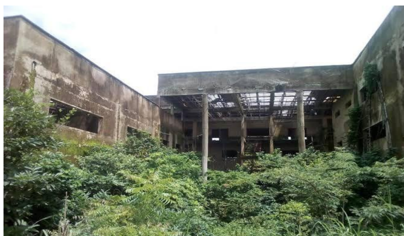
Plate 1: Abandoned Multi-million School Project in Abeokuta.
