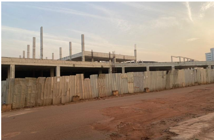
Plate 6: Abandoned Proposed Shoprite Building in Abeokuta. Source: Authors' Field Survey, 2024
