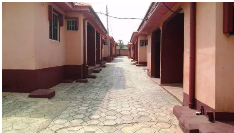
Figure 23: Buildings arranged in blocks
