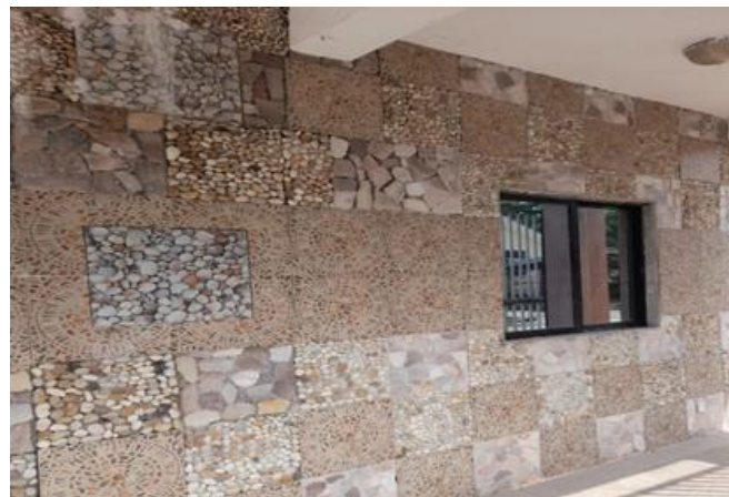
Figure 8 showing the use of stone at Whispering Palms Resort Source: Authors survey
