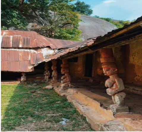
Figure 9a & 9b: Showing statues with different historical meanings used as columns, supporting the weight of the roof of the King Palace sited on the Idanre Hill.
